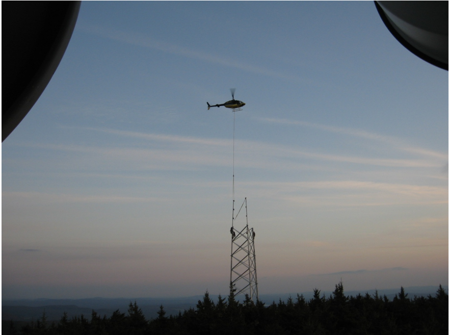
A Helicopter places a section of the new communications tower on the Summit of Belknap Mountain
